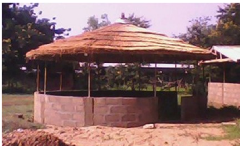
One of two soap shelter buildings, almost completed.
